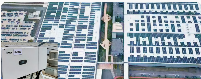
5.99MW ENOVATE Motors EV Manufacturing Base PV Plant in Changsha, China (XG110KTR, XG50KTR)
